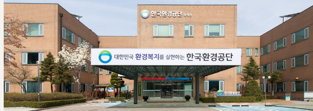
| Front view of K-eco head office |
