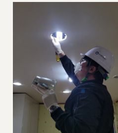
| Asbestos investigation site |
