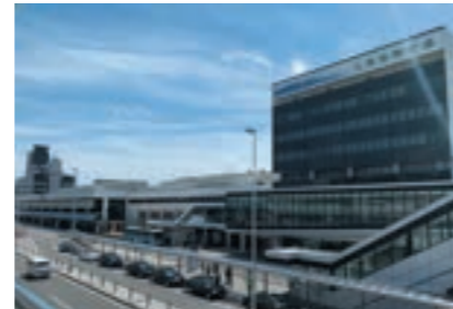
Terminal building renovations at Osaka International Airport (plumbing work)
