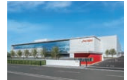
Production equipment for Shiseido Fukuoka Kurume Factory (plumbing work)
