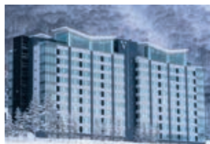
The Vale Rusutsu (Hokkaido) (air conditioning and plumbing works)
