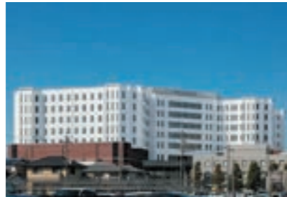
Komaki City Hospital (air conditioning and plumbing works)
