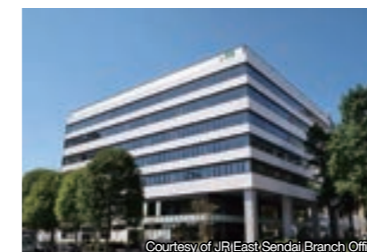
JR East Sendai Branch Office (air conditioning work) Courtesy of JR East Sendai Branch Office
