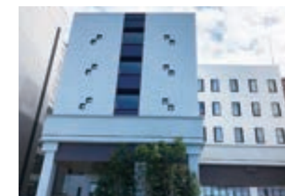
National Center for Geriatrics and Gerontology (Aichi Pref.) (electrical work)
