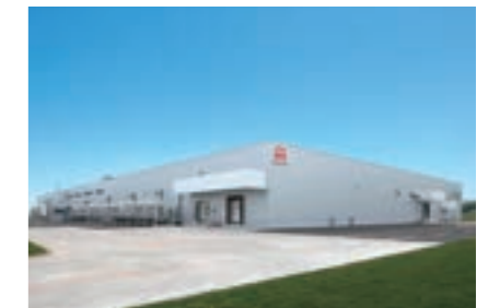
New factory for Nipponham Hokkaido Factory Ltd. (air conditioning and plumbing works)
