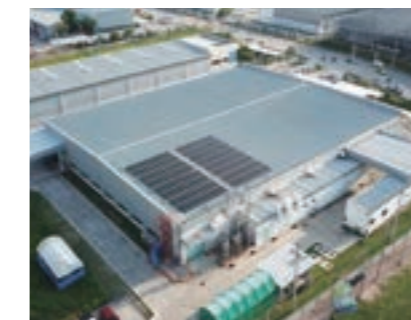
Thailand Solar cells for existing factory (Mie Precision Machining)
