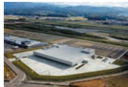
Kawakita Factory, Shinko Chemical (air conditioning and plumbing works)
