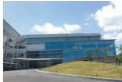
SE1 Building, AGC Yokohama Technical Center (air conditioning and plumbing works)
