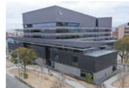
New government office building, Yatsushiro City (air conditioning and plumbing works)
