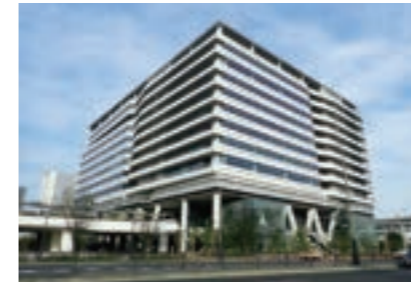
Mebks Toyosu (air conditioning and plumbing works)
