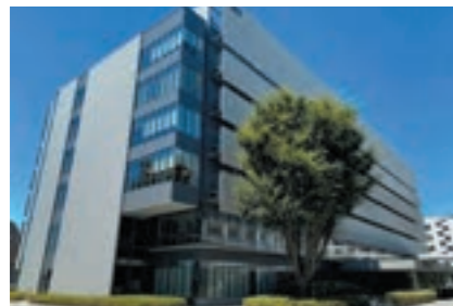
A1 Building, Kitasato University School of Allied Health Sciences (electrical, air conditioning and plumbing works)
