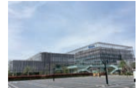
Kurita Innovation Hub (Tokyo) (electrical work)
