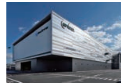
New factory for GS Yuasa (Kyoto Pref.) (plumbing work)
