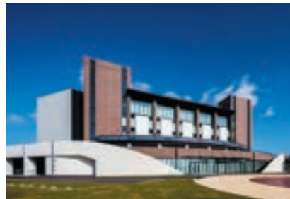
Okinawa Arena (air conditioning work)
