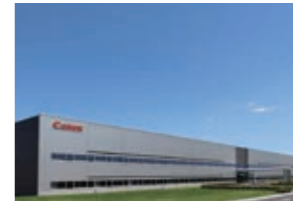
New factory for Canon Mold (Ibaraki Pref.) (electrical work)
