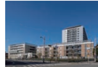
Hyogo Prefectural Harima-Himeji General Medical Center (plumbing work)
