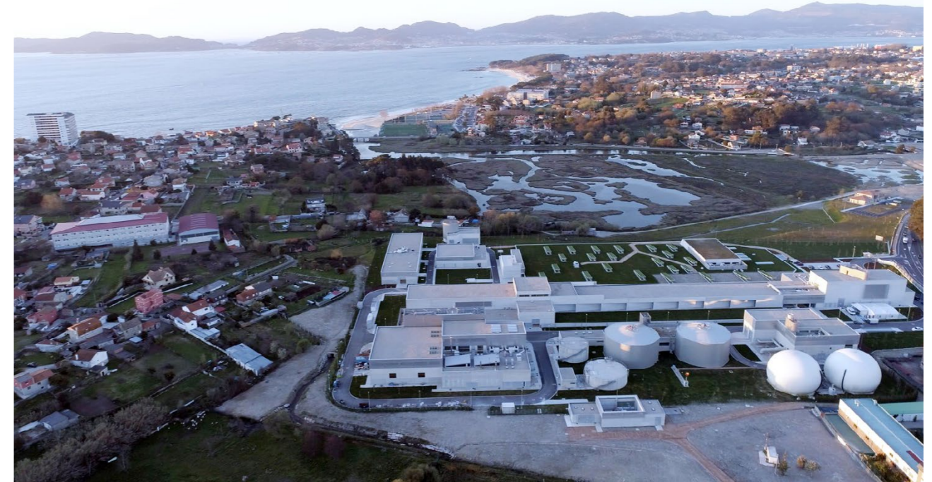
Wastewater Treatment Plant (WWTP) in Lagares, Vigo, Pontevedra, Spain.
