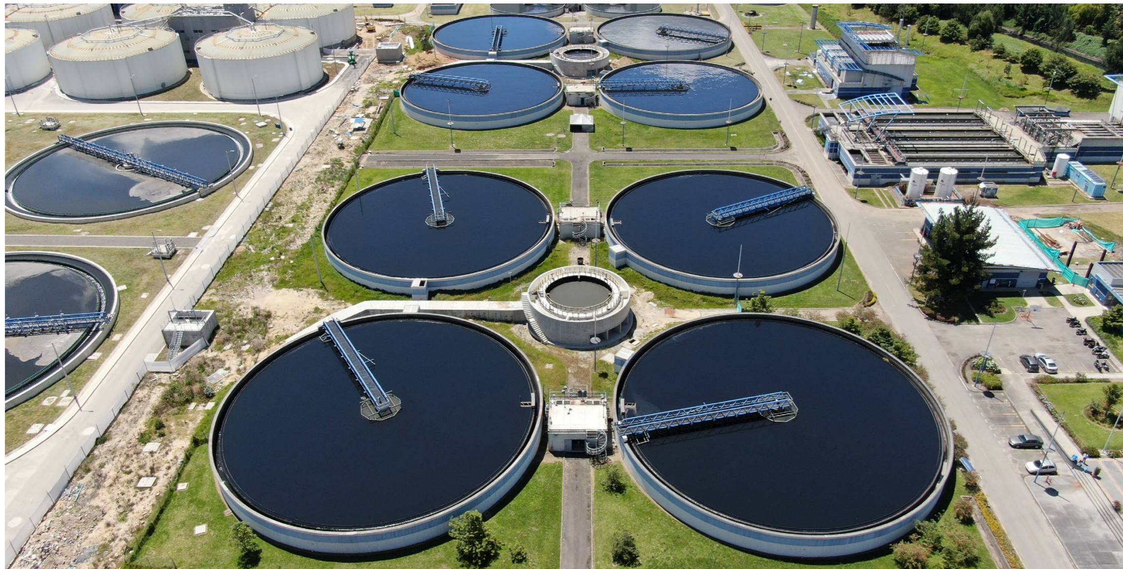
Wastewater Treatment Plant (WWTP) El Salitre, Bogota, Colombia.
