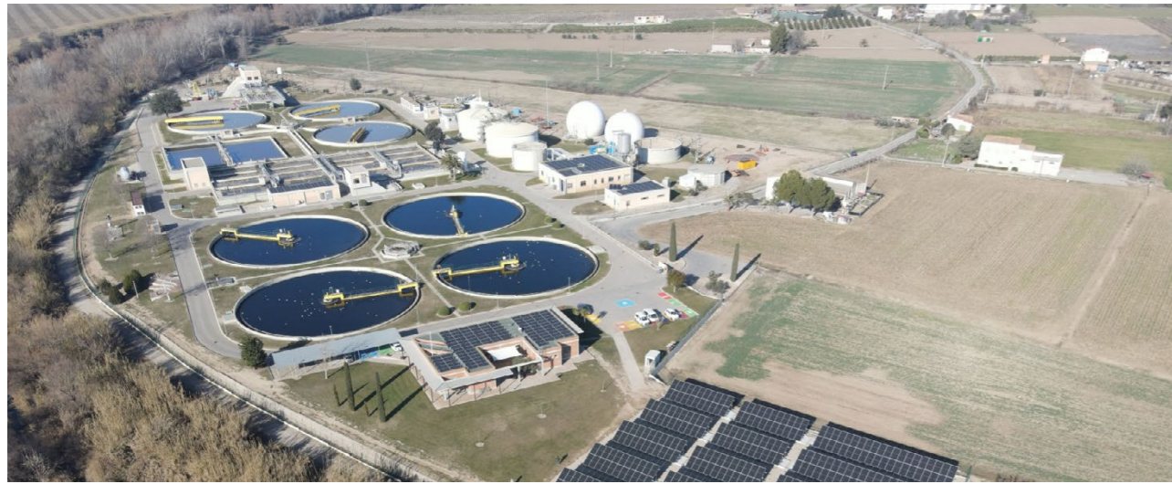
Wastewater Treatment Plant (WWTP) in Lleida, Catalonia, Spain.
