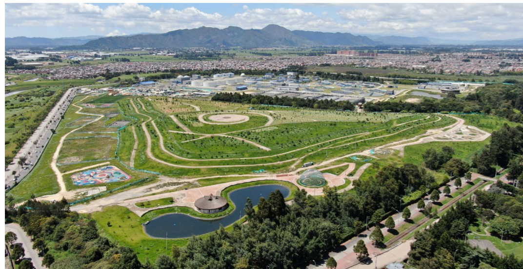
Parque Metropolitano at the Wastewater Treatment Plant, El Salitre, Bogotá, Colombia.
