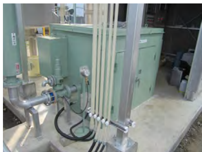
Biological processing facility (aeration blower)
