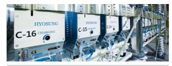
Static Synchronous Compensation (STATCOM) by Hyosung Heavy Industries
