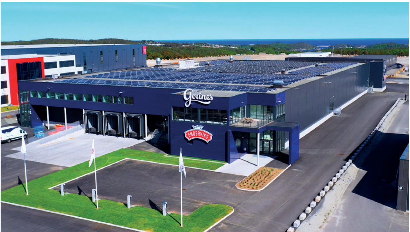
In this building, solar panels and geothermal wells help to ensure sustainable food production, and batteries enable Gorines to store any renewable energy they do not use themselves. That energy can be sold on when grid demand is high.
