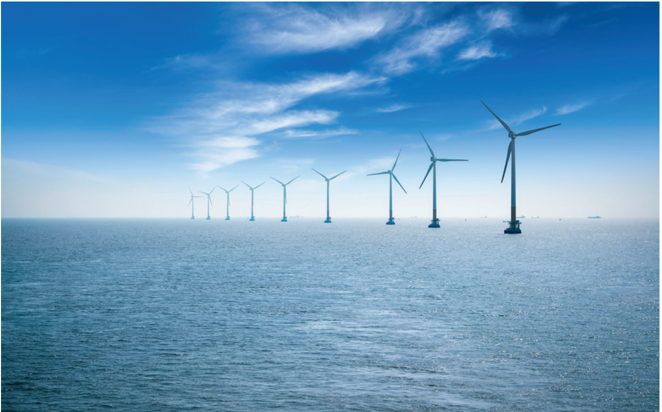
For the competition to develop an offshore wind farm at Utsira Nord, Agder Energi has partnered with Green Investment Group, one of the world's largest investors in and developers of green infrastructure. Diagram: Envato Elements
