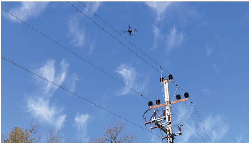
Agder Energi Nett has started using drones to inspect its electrical grid. Compared with helicopters, drones help to reduce CO2 emissions, noise and health and safety risks.
