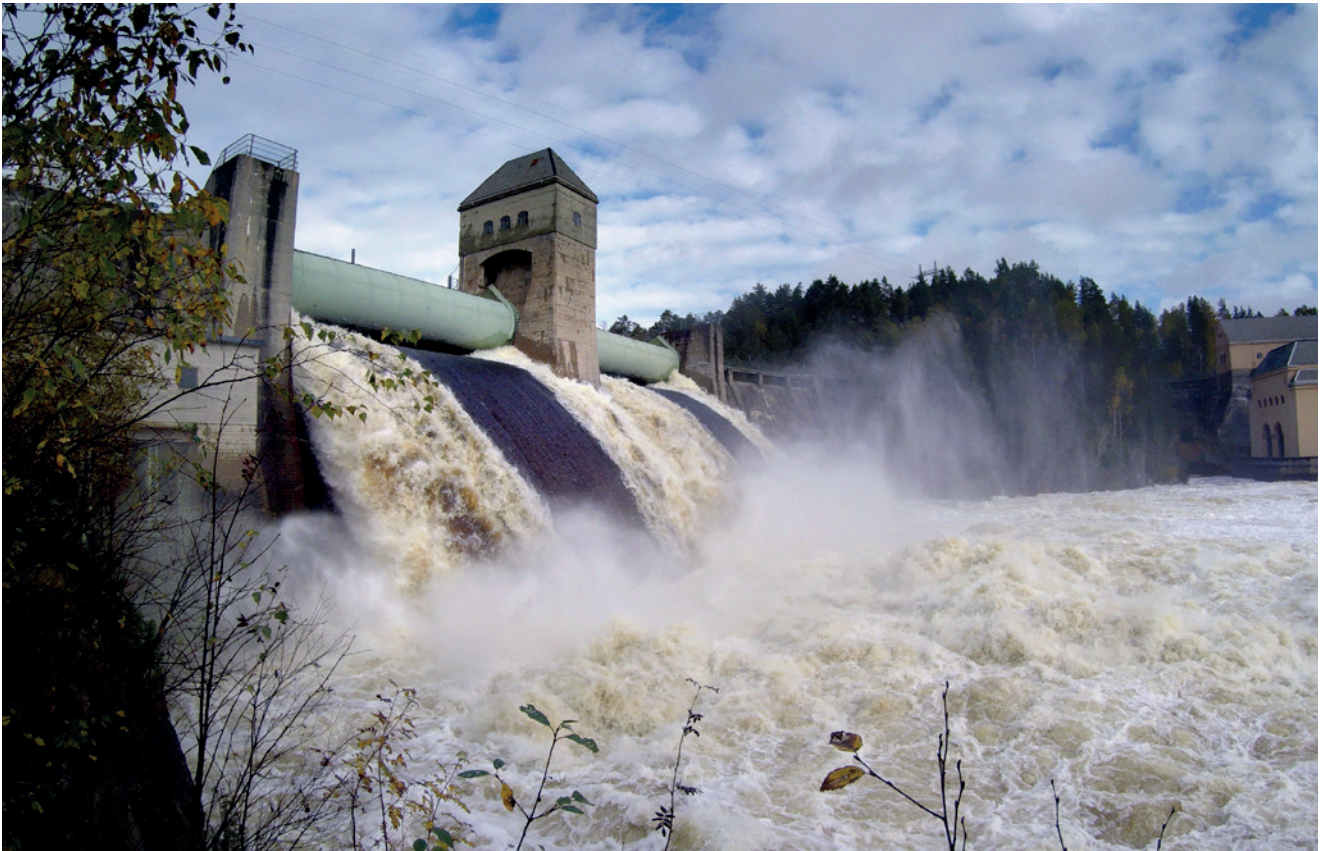
Normally, damming river systems helps to smooth out fluctuations in streamflow, and it can significantly mitigate flooding. The degree of mitigation depends on the amount of water that can be stored in relation to the size of the drainage basin. The picture is from the great flood in October 2017, when large amounts of water flowed out of the dam at Nomeland power plant in Iveland.
