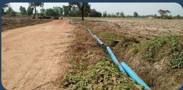
Implementing factory wastewater diversion for agricultural continuity and sustainability project to address agricultural water shortage. Wastewater sewer pipes and pumps have been installed on the farming area of 1,200 rai in Muang district, Udon Thani province. The plan is to install 2,000 meters of sewer pipe, accommodating 100 rai of farming areas, each year
