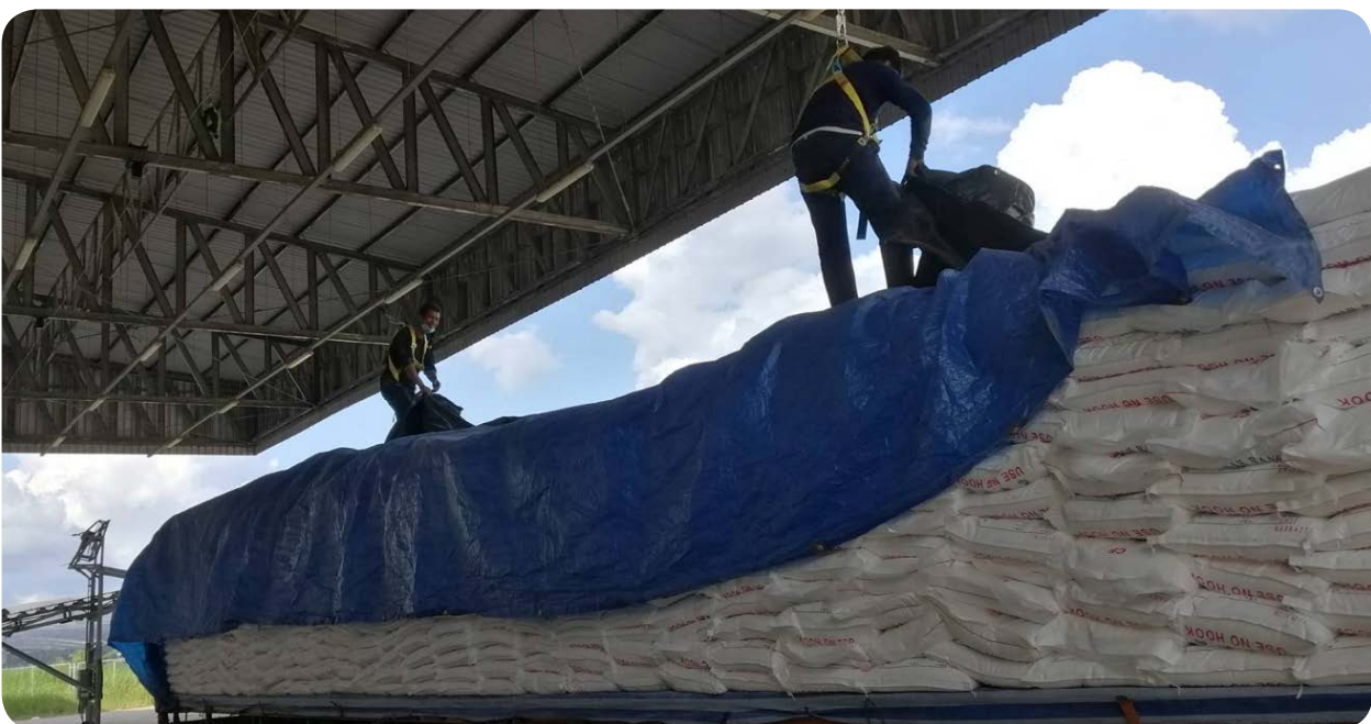
Install a lifeline for working at height to prevent dangerous accidents during work.
