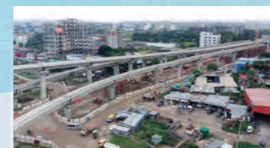
Bangladesh Dhaka Mass Rapid Transit Development Project
