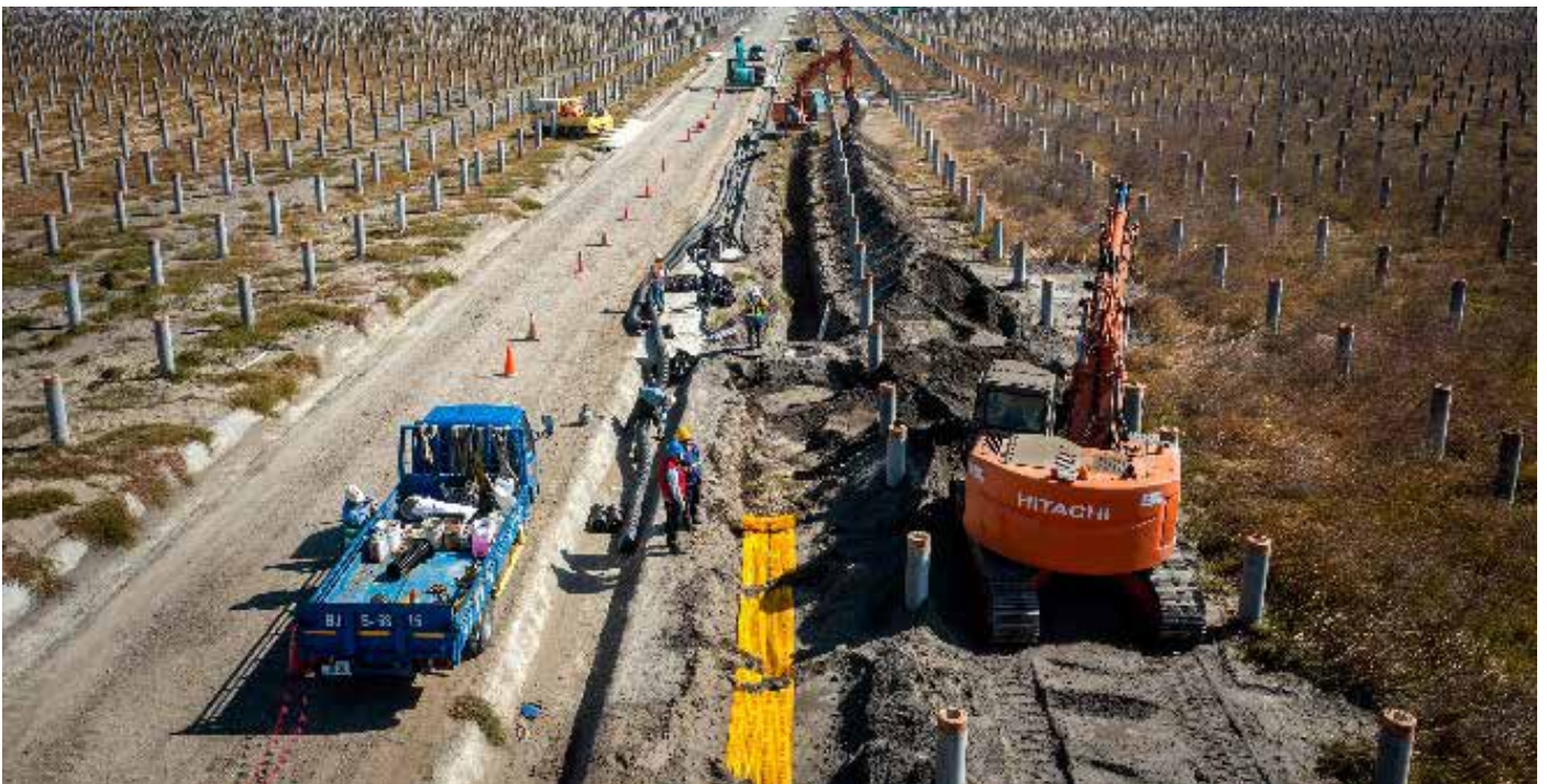
Construction of drainage canal
