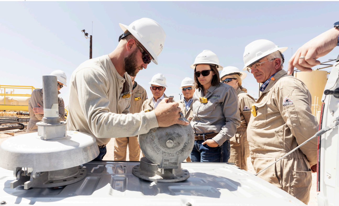
Demonstration of improved thief hatch design (left) vs old (right) to mitigate air emissions.
