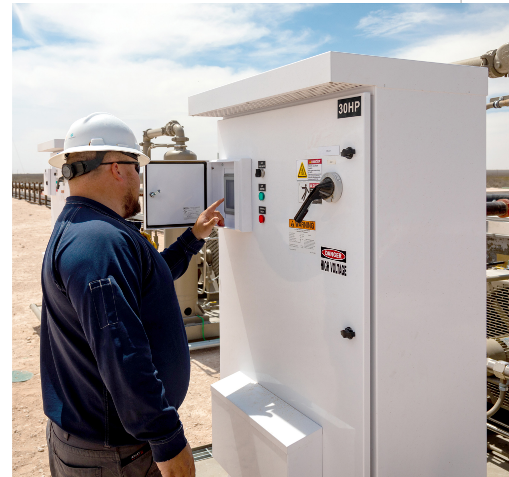
Vapor recovery unit control panel.
