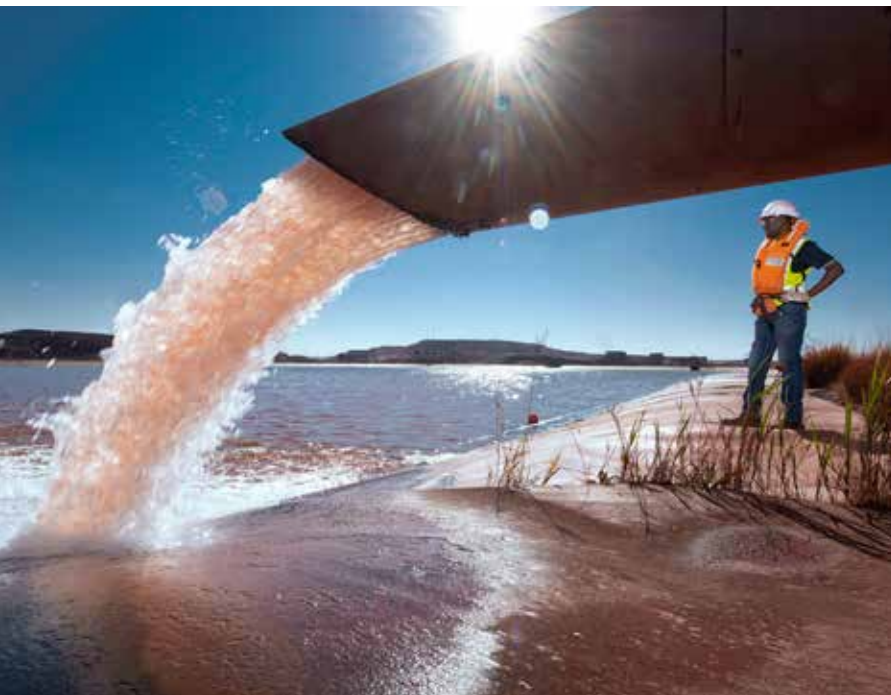
▲ Environmental advisor Andrew Nkhoma at the return-water dam at Sishen, which has been expanded to twice the capacity of the original dam. The dam receives stormwater from the mine's eastern and western sumps and supplies it back to the processing plant, thereby reducing the mine's use of fresh water.
