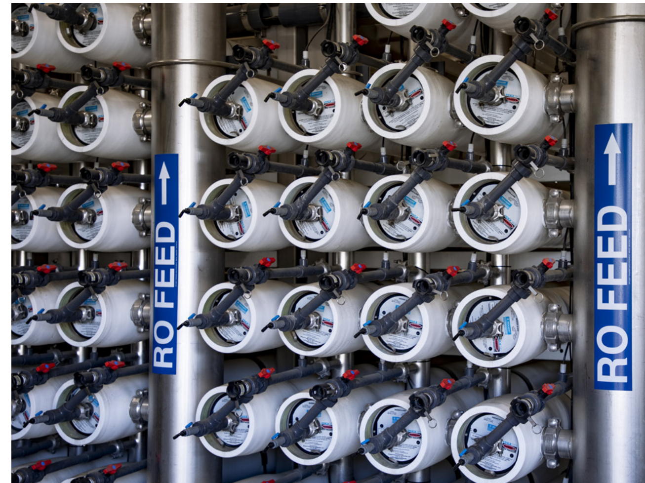
Used in conjunction with FILMTEC™ reverse osmosis (RO) membranes, B-Free™ products are helping DuPont's customers meet their sustainability goals by mitigating the challenges of biofouling and extending the life of the membranes to purify water.
