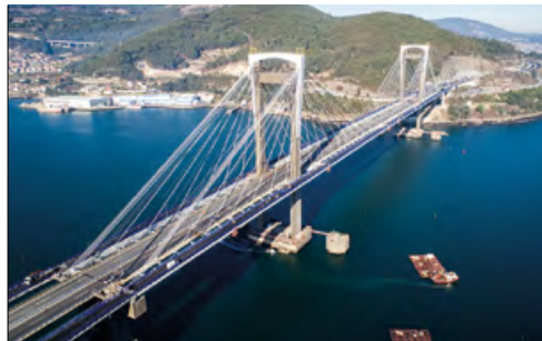
Rande Bridge, Spain
