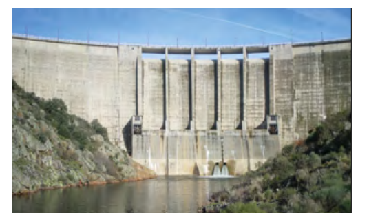
Iruña dam. Salamanca, Spain
