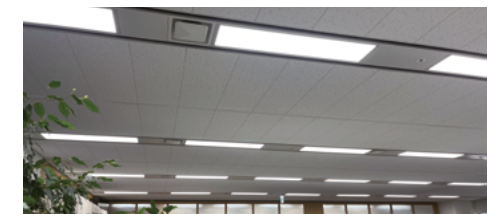
Installation of LED lights in the office
