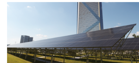
Renewable power generation facilities (Solar)
