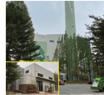
Site of power generation utilizing remaining heat of incinerators after use.
