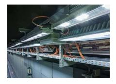
box translates the setpoint into a defined drive signal that is forwarded to the light drivers. Twelve lights are specified per driver box for the interior zone lighting in the tunnel. A driver box for three lights is employed for the reinforcement lighting at the tunnel entrances. The controller works bidirectionally, so it also receives feedback from the driver boxes, such as current values, status reports, and warnings.
