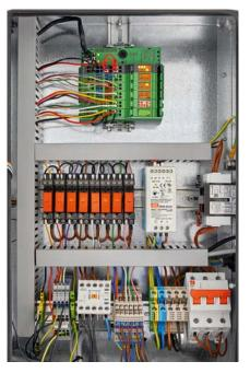
but also reliable system operation. The master controller constantly measures the current wind speed using a wind sensor. If the wind loads are too high, the controllers receive the command to move the trackers out of the wind. This ensures that the photovoltaic modules do not become damaged.
