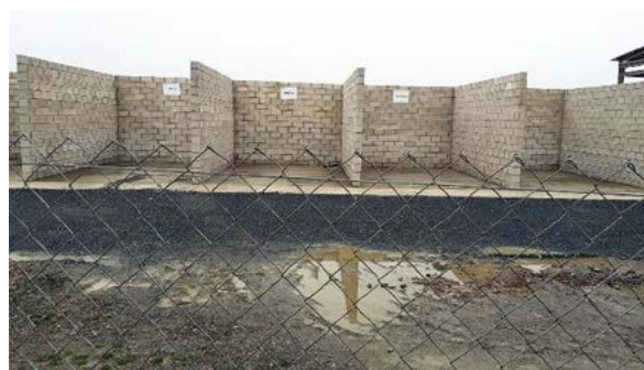
Non-hazardous waste park built in 2021 in Proyecto Riotinto
