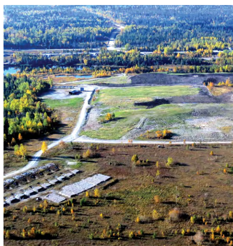
Hemlo site reclamation
