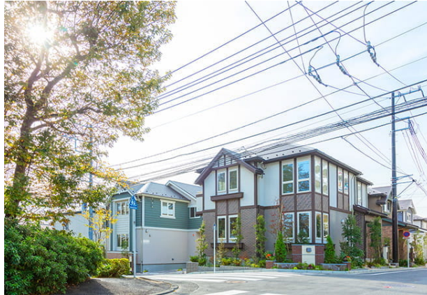
Exterior of The Parkhouse Stage Higashitotsuka using ENE-FARM for all homes
