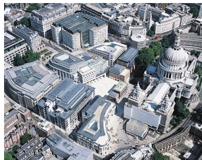
Aerial photo (the property is the square building on the lower left of the square)
