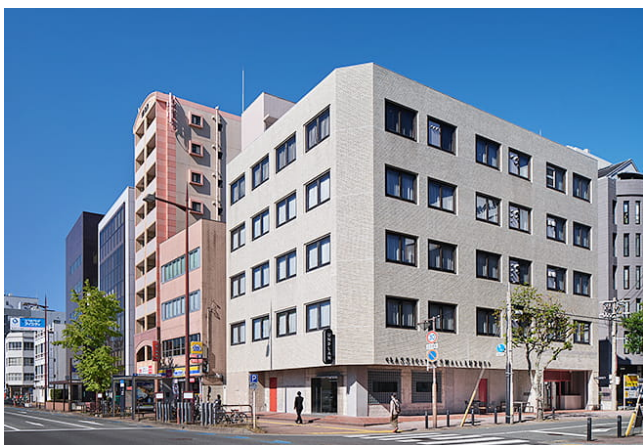
Building exterior after renovation
