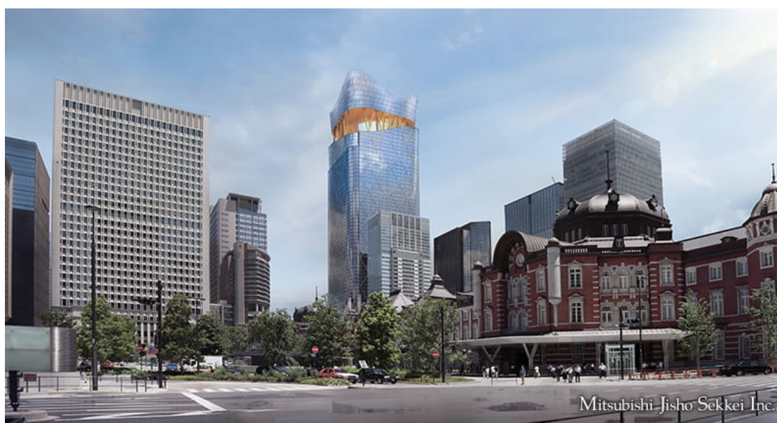
A rendering of TOKYO TORCH overall at the time of its opening as seen from the Marunouchi side of JR Tokyo Station
