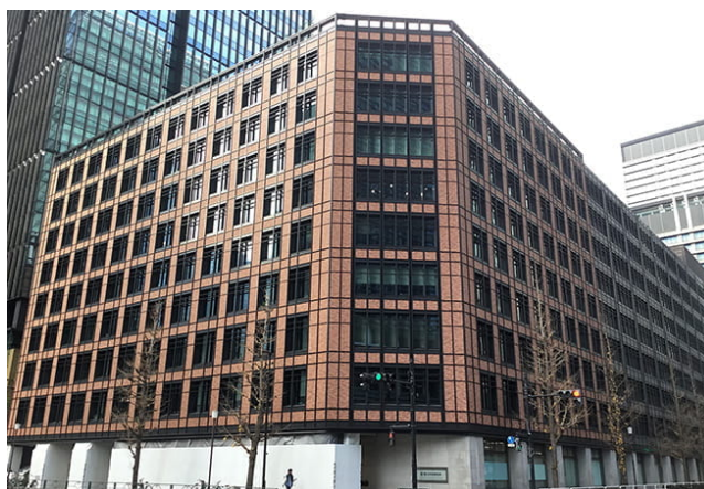
Otemachi Building after renovation
