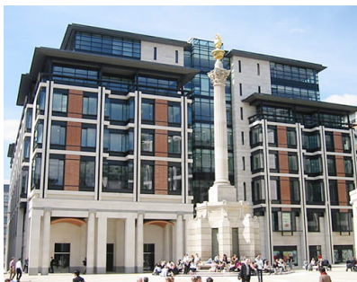
Photo from the building front
