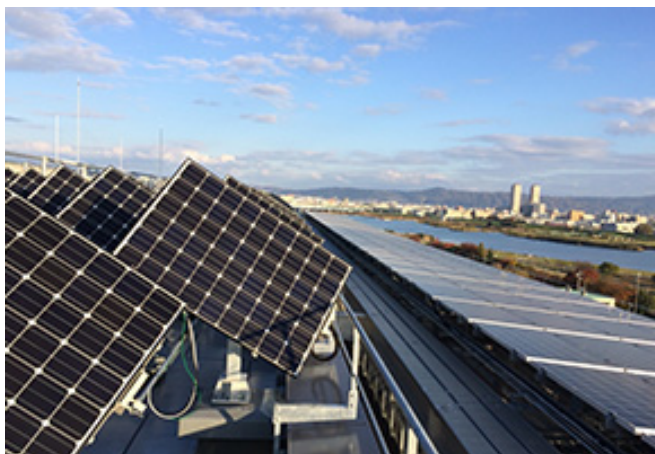
Solar power generation system has panels that move to track the sun's position
