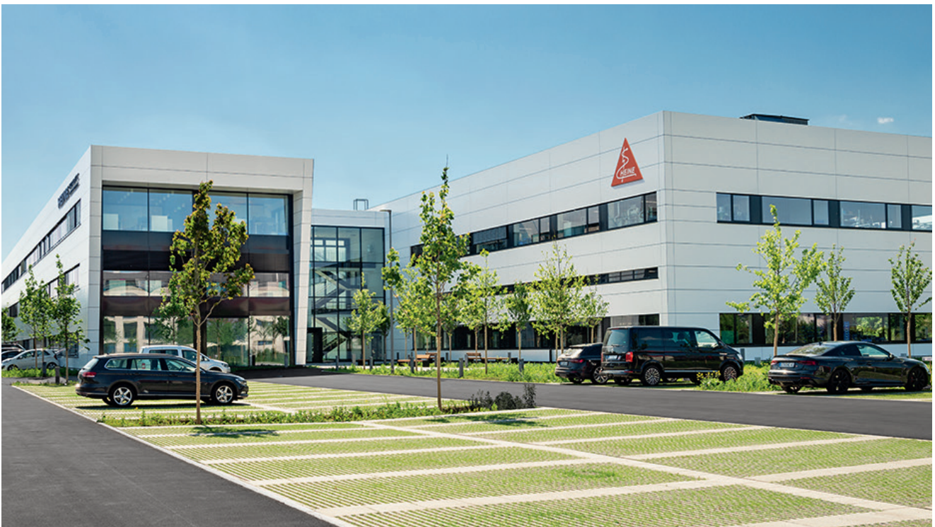
The new HEINE company building in Gilching: On the left the 3-storey administration building, on the right the production building.
