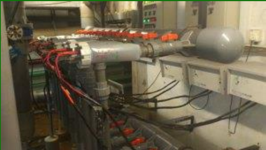
Swimming pool ionization treatment systems
