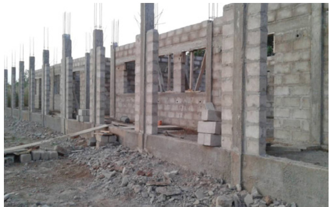
Building a kindergarten in Burkina Faso.
