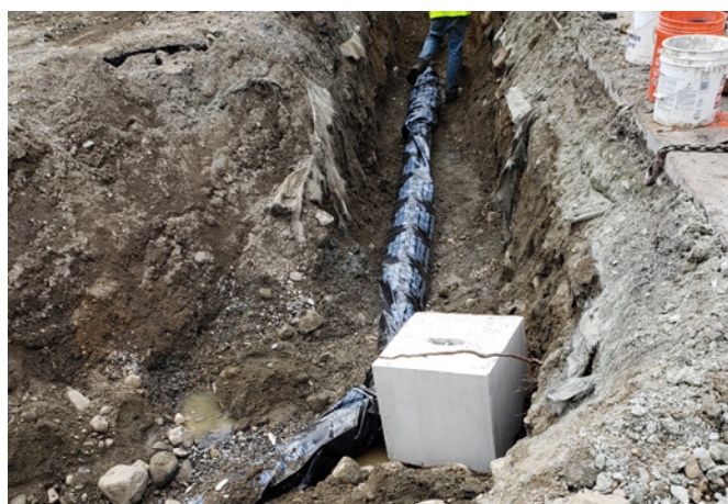
Clean water lines in Bedford.
