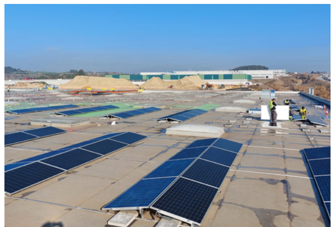
Solar panels being installed in a Werfen facility in Spain in 2021.
