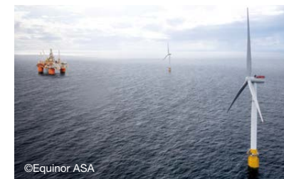
■ Floating wind turbines feeding renewable energy to an offshore oil field
