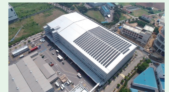
Solar Power Plant in Pyeongtaek
