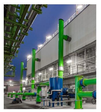
Wesseling (Germany): A cooling tower made of glass-fiber-reinforced plastic reduces the temperature of cooling water after use. Some of the water can be re-used in the cooling system.
