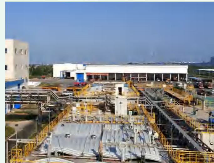
▲ Wastewater treatment of the factory
