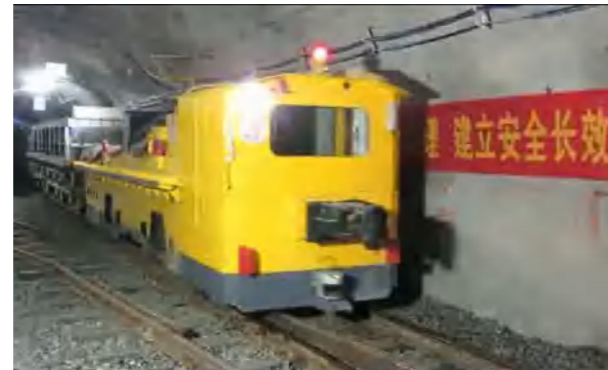
▲ Unmanned electric locomotive underground the mine
