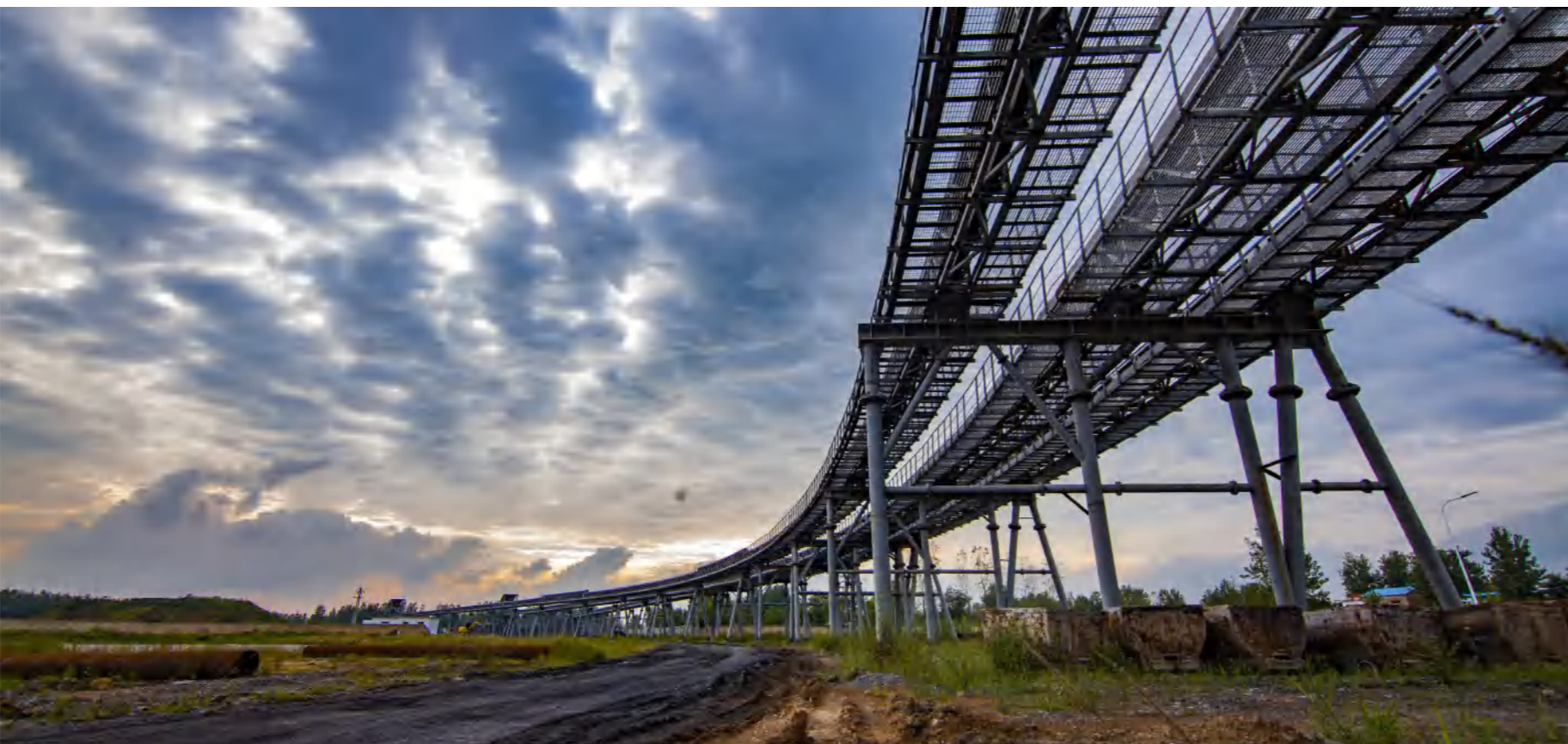
▲ DG250 pipe belt conveyor of Zhangzhuang Mine
