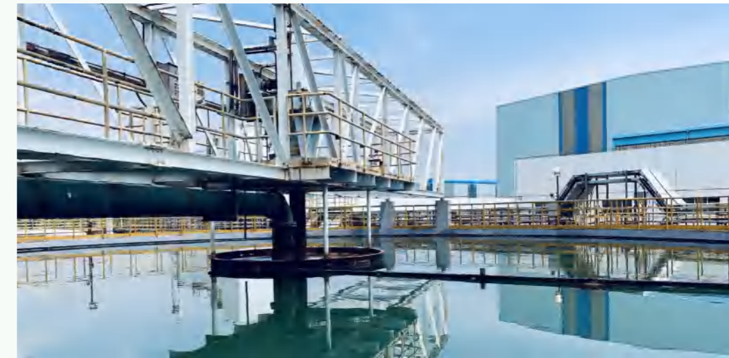
▲ Cold rolling wastewater treatment
