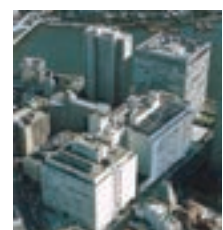
1973 Tokyo Dia Building
