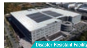
November 2019 Completed Seishin Distribution Center Phase 2 Building in Kobe.
