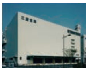
Chuo Futo Warehouse, Fukuoka Branch
