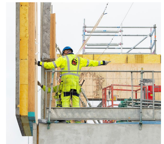
Hybrid elements are being used in the construction of Metsä Fibre's Rauma sawmill.
