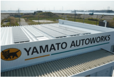
Yamato Autoworks Co., Ltd. plant with low environmental impact (Super Works Nagoya) The Super Works Nagoya is a low-carbon plant that uses solar power generation and energy storage systems, with LED lighting throughout.
