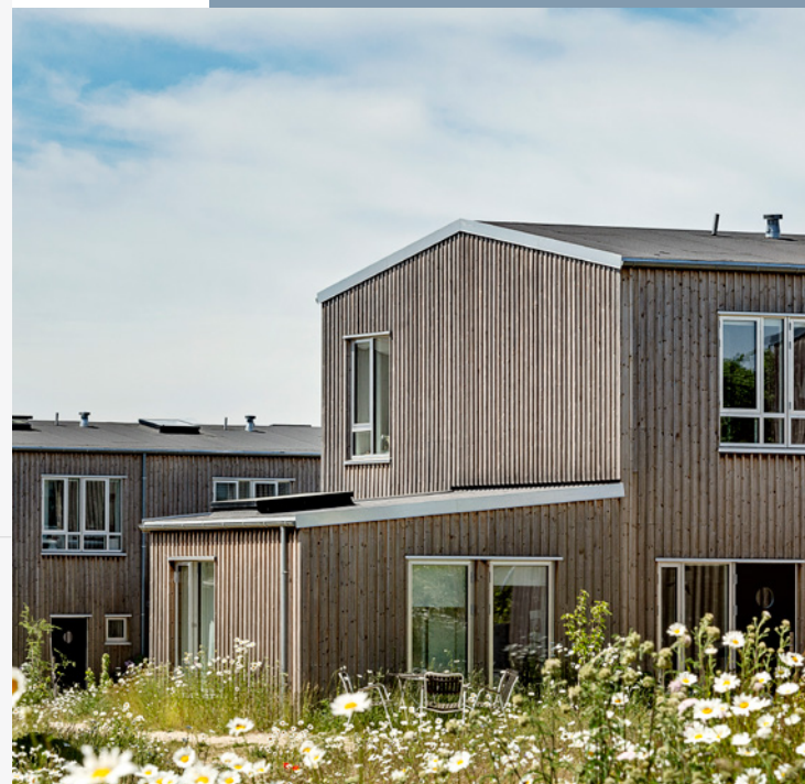
< SKRÅNINGEN II On Skråningen II in Lejre, Scandi Byg has erected 46 wood-clad houses in materials with the Nordic Swan Ecolabel.
