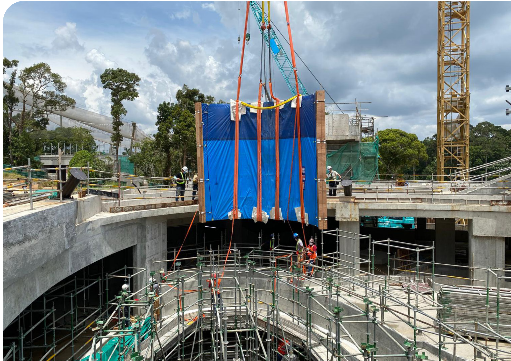
ABOVE: Installation of one of the acrylic sheets at Penguin Cove in the new bird park.
