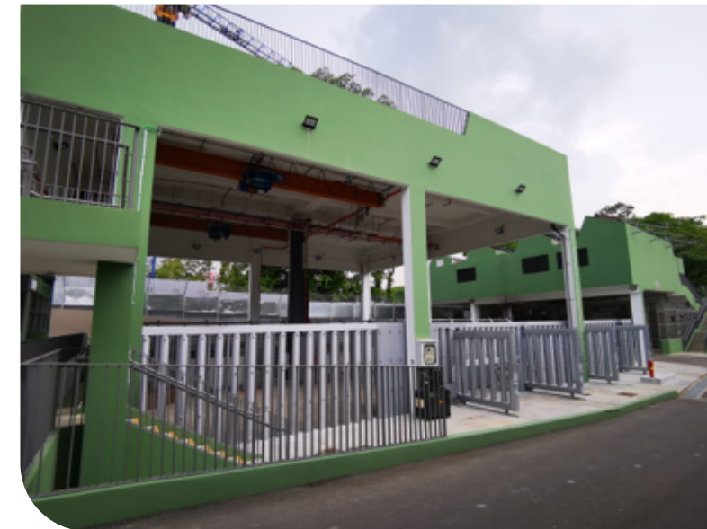
RIGHT: With a size of 2,320 sqm, the new animal quarantine building prepares us well in handling the anticipated increase in the number of quarantine animals as the new parks open progressively.
