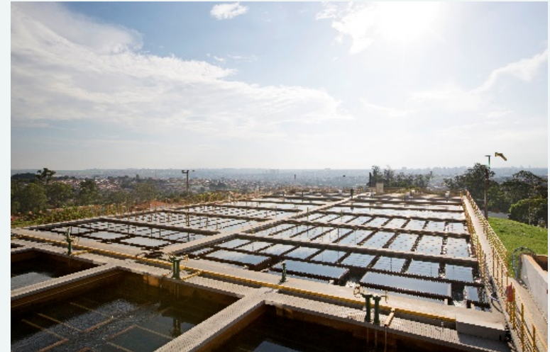
Water treatment plant in the State of São Paulo
