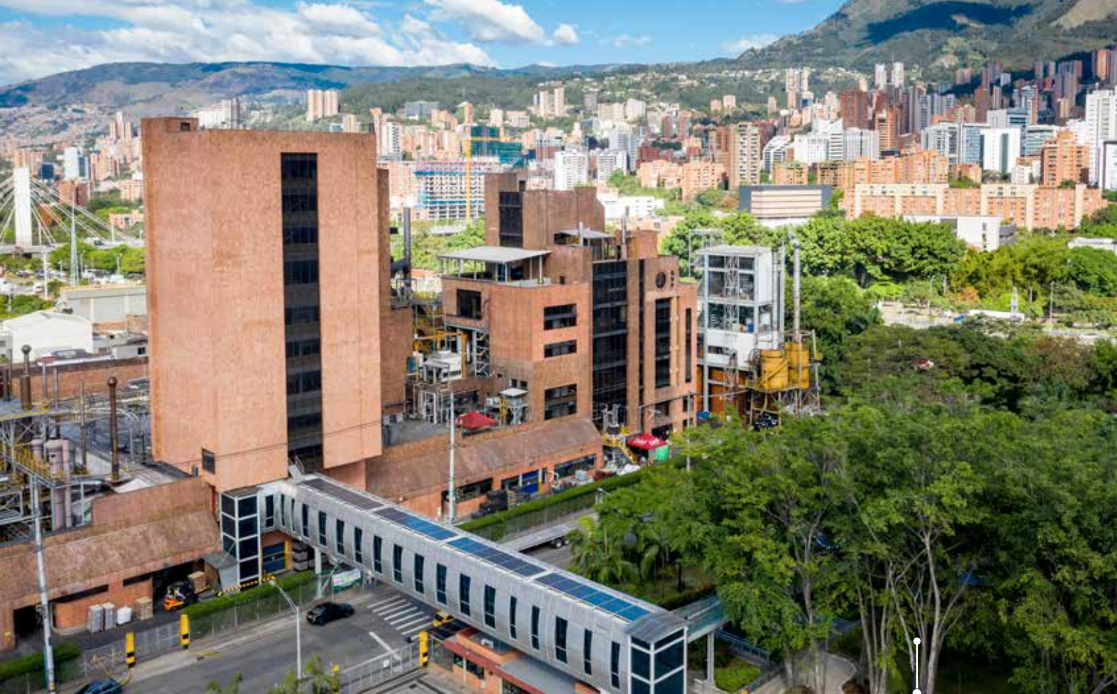
Solar panels installed at the Coffee Business production plant in Medellín, Colombia.
