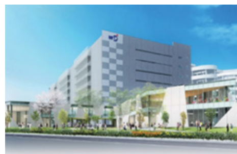
Exterior perspective, Mitsui Fudosan Logistics Park Funabashi
