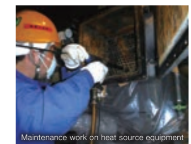
Maintenance work on heat source equipment
