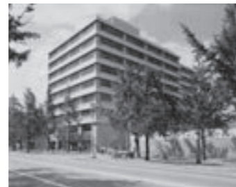
Keihanshin Kawaramachi Building (Completed in 1962)
