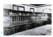
Magnetic parallel multiple telephone switchboard
