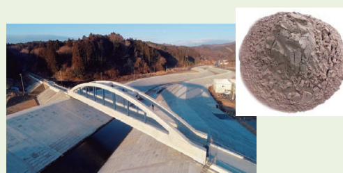
CfFA® was used in bridge beams, arches and vertical supports at the JR Kesennuma Line Sakuragawa Bridge on the JR Kesennuma Line (Minamisanriku Town, Motoyoshi District, Miyagi Prefecture)
