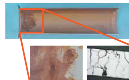
Example of corrosion analysis (Piping sampling inspection)
