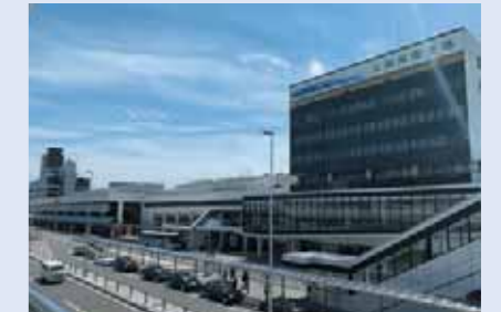
Terminal building renovations at Osaka International Airport (plumbing installation)
