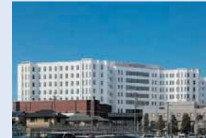
Komaki City Hospital (air conditioning and plumbing installations)
