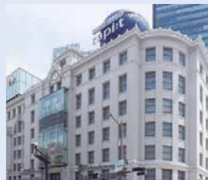
Nankai Terminal Building Nankai Electric Railway Co., Ltd. (electrical installation)
