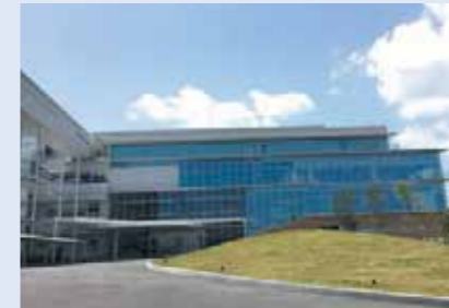
SE1 Building, AGC Yokohama Technical Center (air conditioning and plumbing installations)
