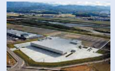
Kawakita Factory, Shinko Chemical (air conditioning and plumbing installations)
