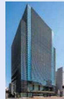
Head Office Building, Hirogin Holdings (air conditioning installation)
