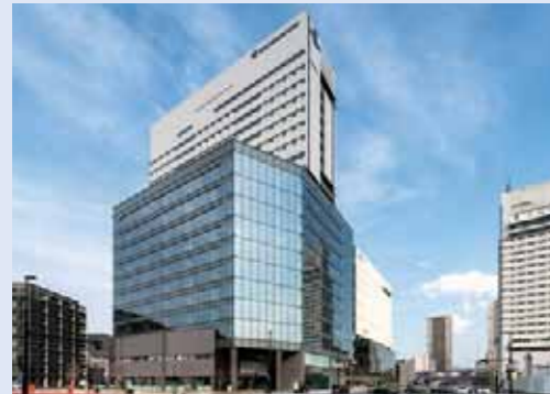
GRANODE Hiroshima (electrical, air conditioning and plumbing installations)
