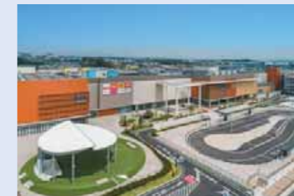
LaLaport Aichi Togo (electrical installation)
