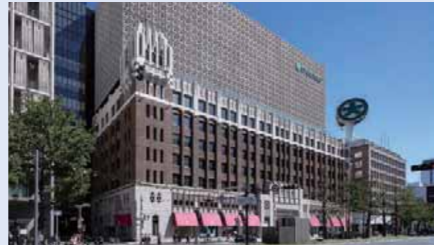
Main Building, Daimaru Shinsaibashi Store (electrical installation)
