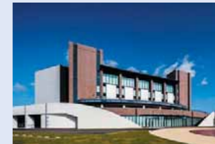
Okinawa Arena (air conditioning installation)
