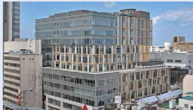
Furumachi Refuru (air conditioning and plumbing installations)
