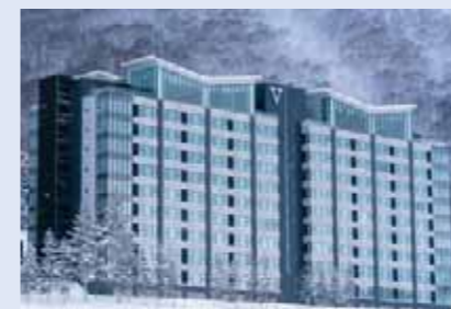
The Vale Rusutsu (air conditioning and plumbing installations)
