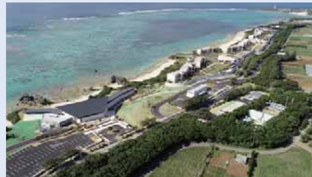
HOSHINOYA Okinawa (air conditioning and plumbing installations)
