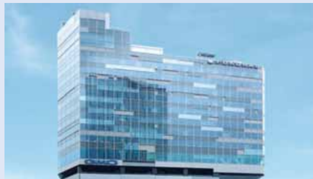
SHIBUYA FUKURAS (air conditioning and plumbing installations)
