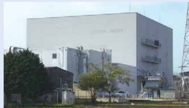
Headquarters Plant, Tokai Capsule Co., Ltd. (air conditioning and plumbing installations)
