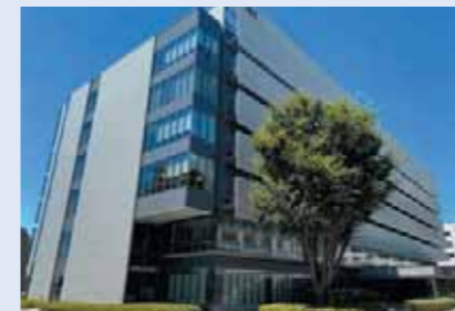
A1 Building, Kitasato University School of Allied Health Sciences (electrical, air conditioning and plumbing installations)
