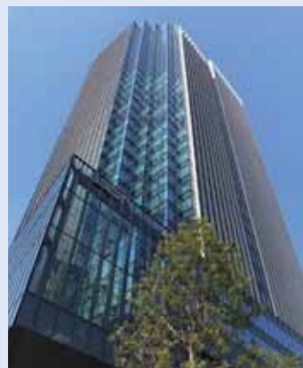
CO·MO·RE YOTSUYA (air conditioning installation)
