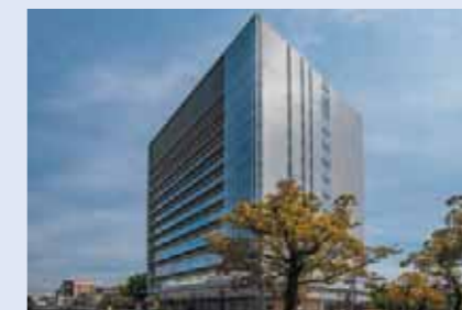
Government Office Building No. 2, Nishinomiya City (air conditioning and plumbing installations)
