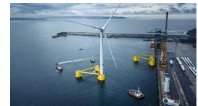
洋上風力発電向け浮体基礎システム (Photo courtesy of Principle Power. Artist: DOCK90)
