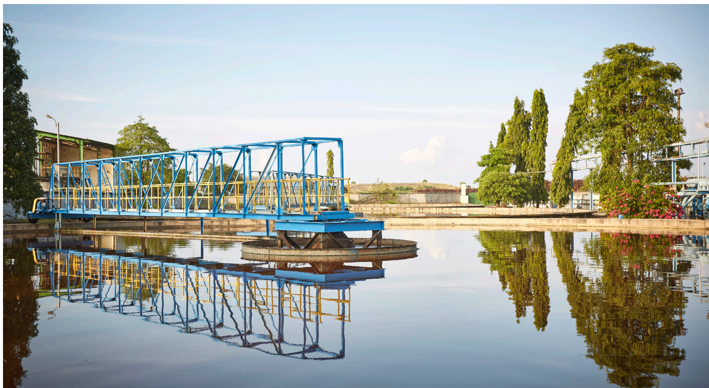
Waste water treatment plant Fasilitas pengelolaan limbah cair
