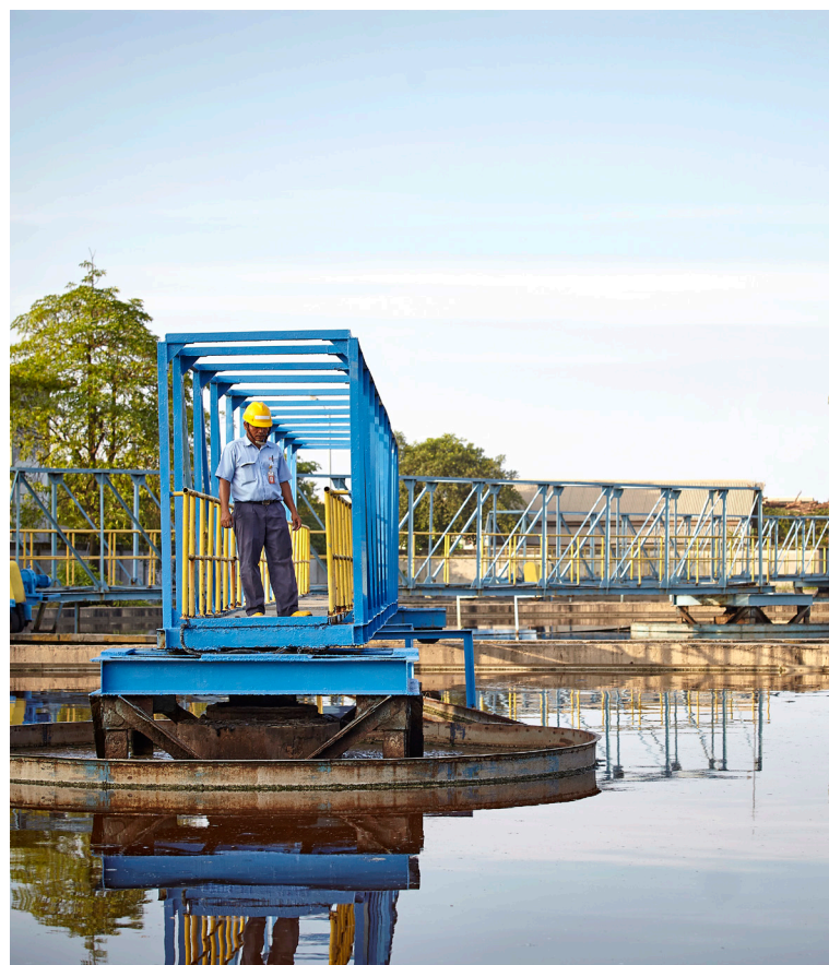
Waste water treatment plant Fasilitas pengelolaan limbah cair
