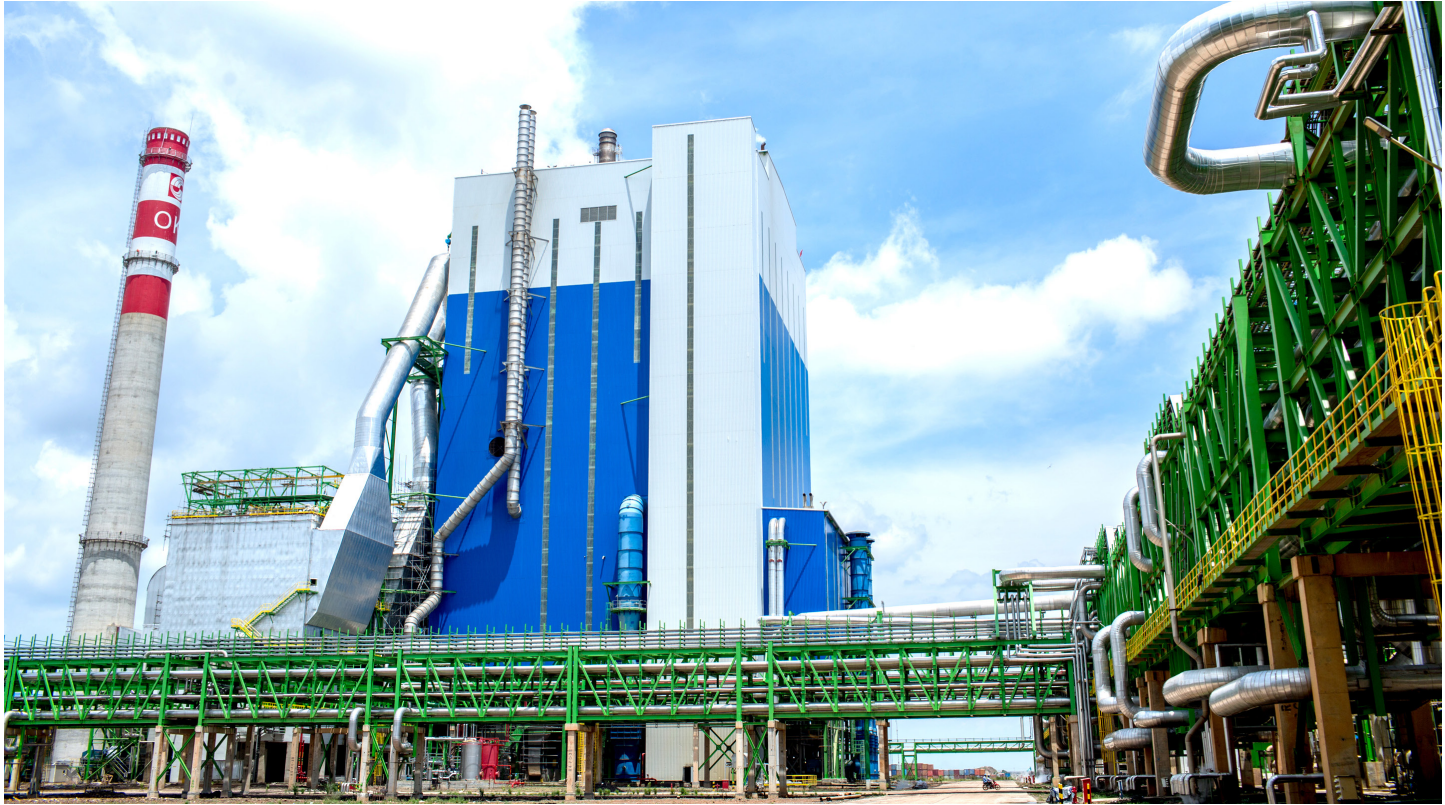
Recovery boiler, generating renewable energy Recovery boiler, menghasilkan energi terbarukan
