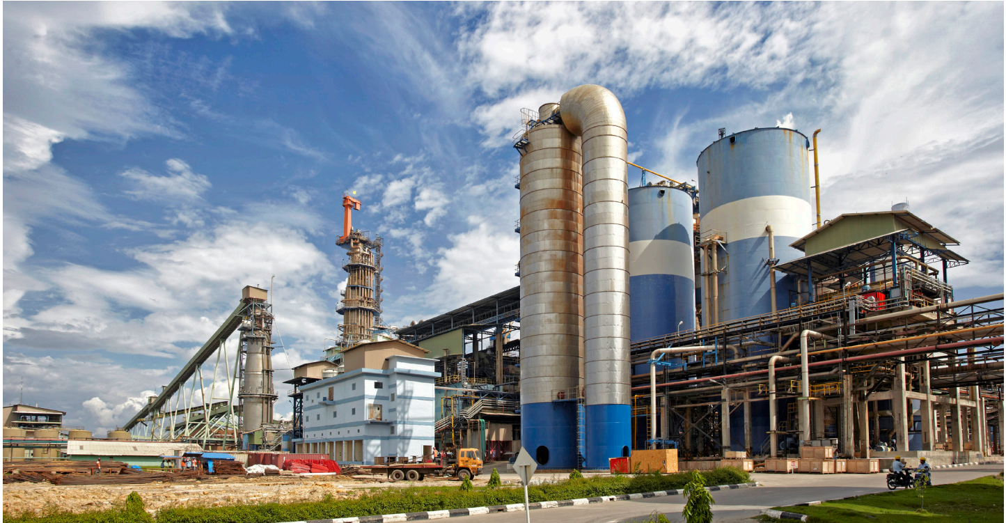
Pulp production facility at Lontar Papyrus Pabrik produksi pulp di Lontar Papyrus
