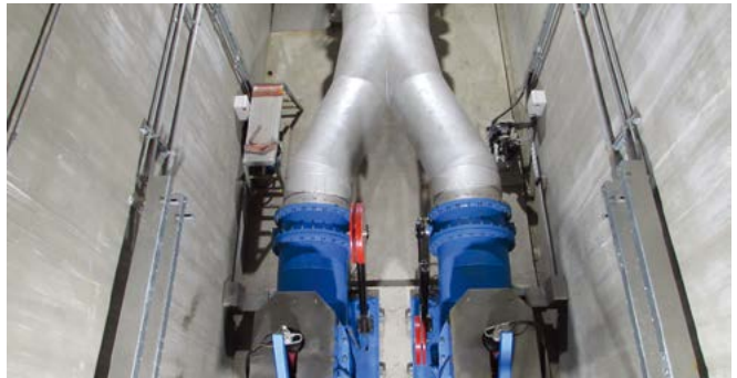
Installation of small hydro-power generator in the basement near the Icheon business site's wastewater treatment plant
