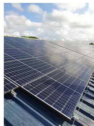
New solar panels installed on the roofs of the fermentation facility
