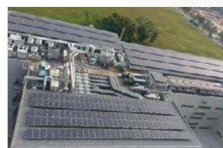
Roof of the Factory Building
