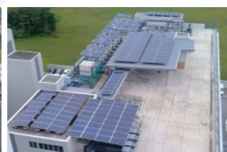
Roof of the Administrative Building
