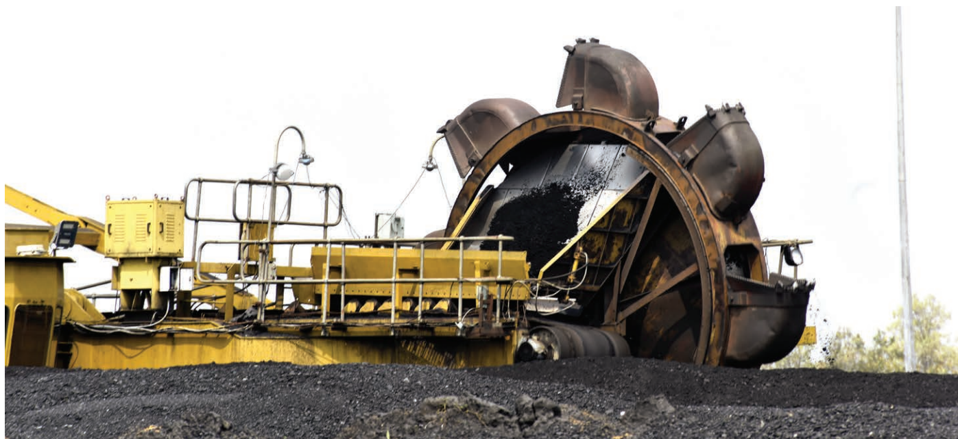
Coal Yard at our Thermal Power Plant
