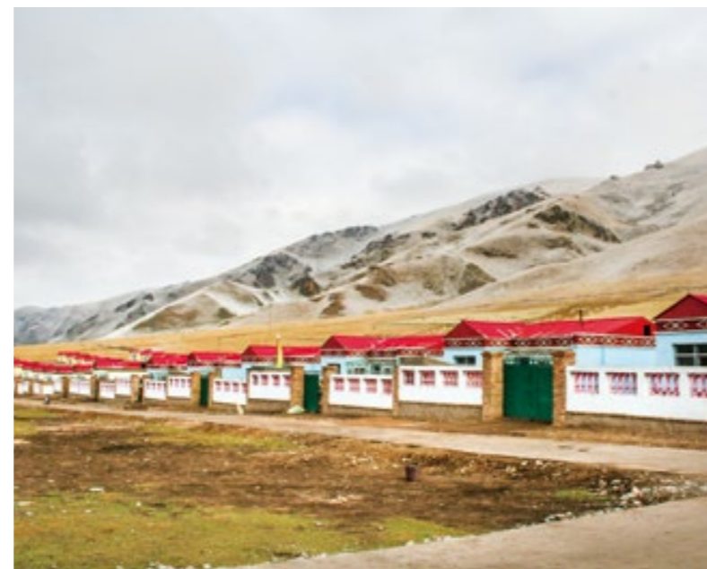
Construction of housing for herdsmen
