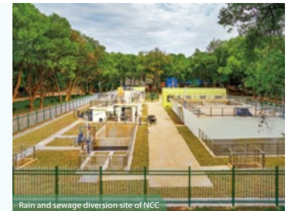
Rain and sewage diversion site of NCC
