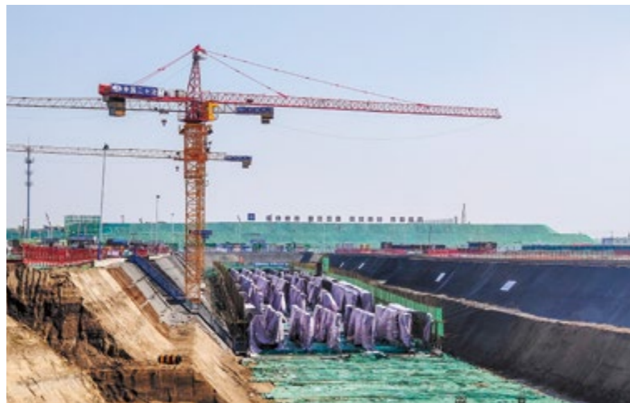
Construction site of Rongdong AF community project in Xiong'an New Area
