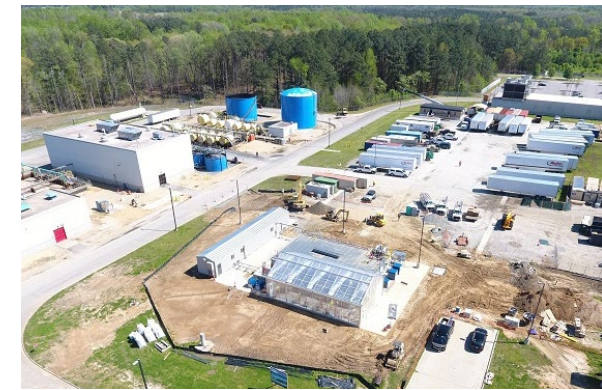
Cummins employees (left) at the company's engine plant in Rocky Mount, North Carolina (U.S.), officially launch the plant's Water Hub (above) in 2020. It uses a variety of treatment technologies including hydroponics to return millions of gallons of water to the plant annually for non-potable uses.
