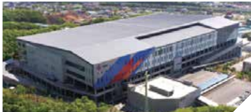
Gonjiam Mega Hub Terminal
