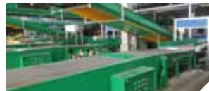
Installation of protective covers
