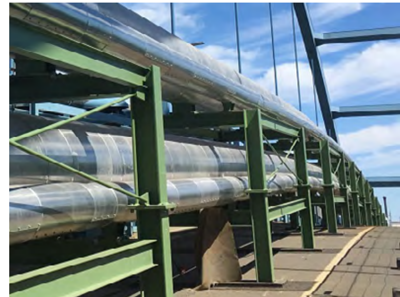
Industrial heat from the Hamburg site is used to supply heat to the HafenCity East and Rothenburgsort districts
