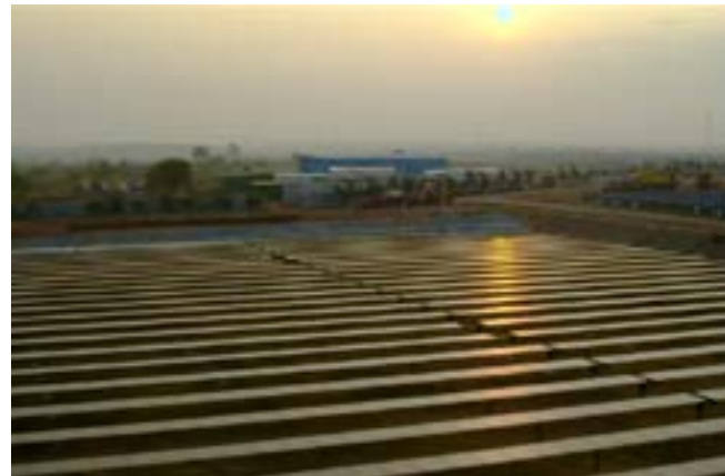
Solar plant in Sira, Karnataka
