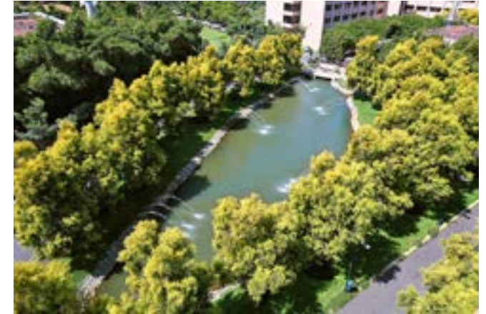
Rainwater harvesting pond in Infosys, Bengaluru campus
