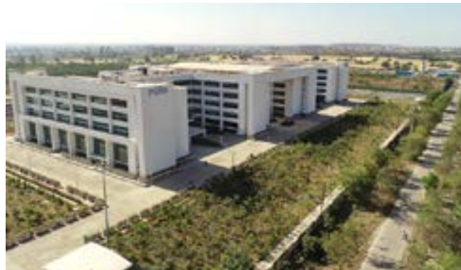
Infosys, Indore SDB – LEED Platinum certified building
