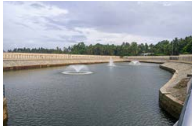
Rainwater harvesting pond in Infosys, Thiruvananthapuram campus
